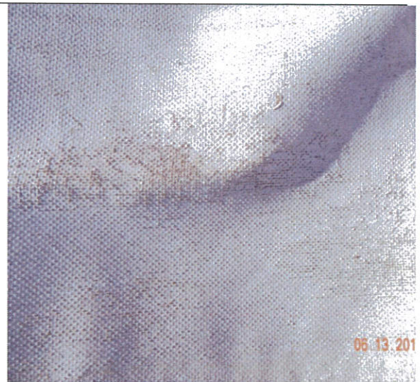
33b-west-P1716_20170613_JG01-033 Example of fabric scrim visible
