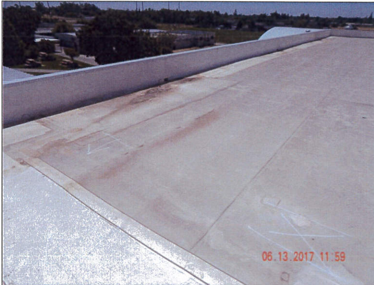
39a-east-P1716_20170613_JG01-104 Markings of moisture locations on east gym section
