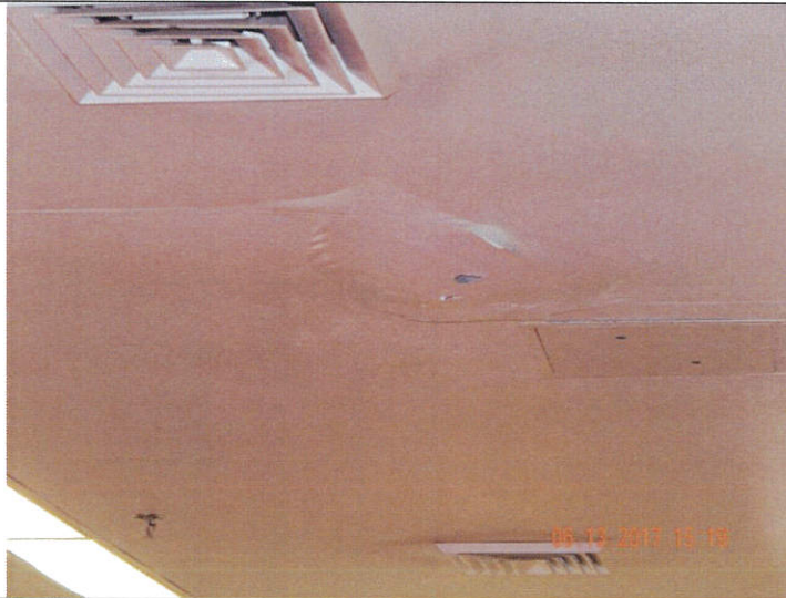
21-P1716_20170613_JG01-190 Locker room with signs of roof leakage
