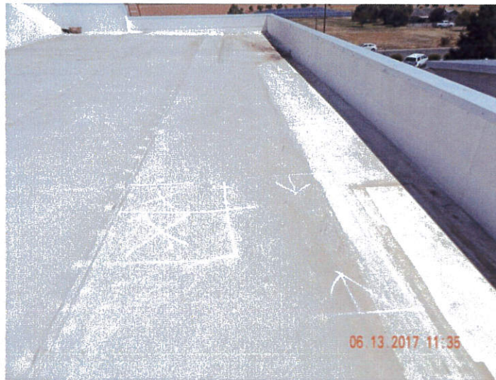
43-east-P1716_20170613_JG01-075 Examples of positive reading locations on East Gym
